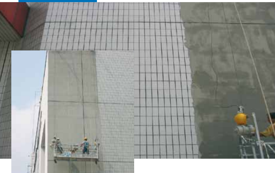
Applying Planitop 200 on ceramic substrate
