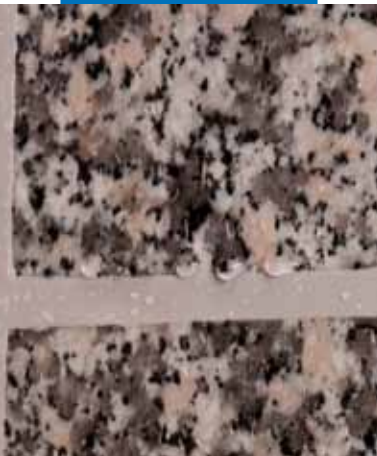
Sealing an external stone dressing
