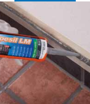
Sealing an internal stone dressing
