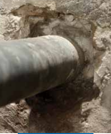
Demolition of the structure around a pipe
