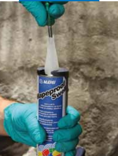
Piercing the protective membrane on the Mapeproof Swell tube
