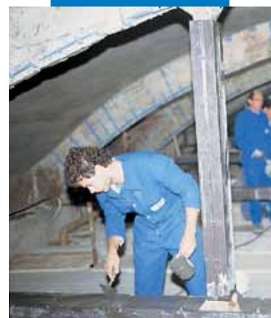
Pouring Mapegrout Hi-Flow into metal formwork
