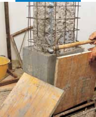
Removing wooden formwork
