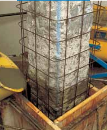
Pouring into a formwork
