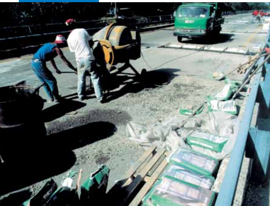
Reforming road joints
