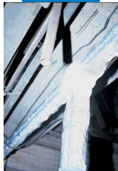
Deteriorated concrete structure
