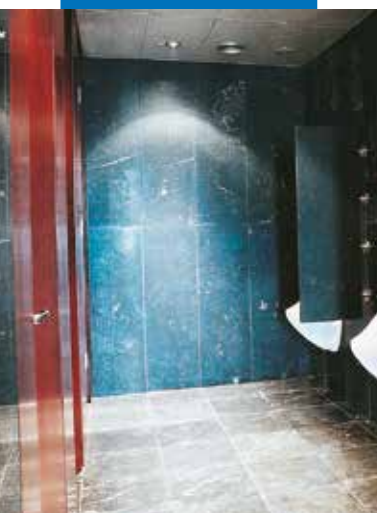
An example of the installation of marble to walls with Keraquick S1 - Feuchtwangen casinò bathroom (Germany)
