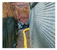
**Platon DOUBLE DRAIN** must be installed over a primary membrane, such as brushed on bitumen coatings. Fix **Platon DOUBLE DRAIN** along the top edge above the primary membrane, with **Platon DOUBLE DRAIN** cramps at 250mm centres. Overlap vertical joints by 120mm and horizontal joints by 120mm. Filter fabric can be pulled back for successive overlap of the membrane and filter fabric.
